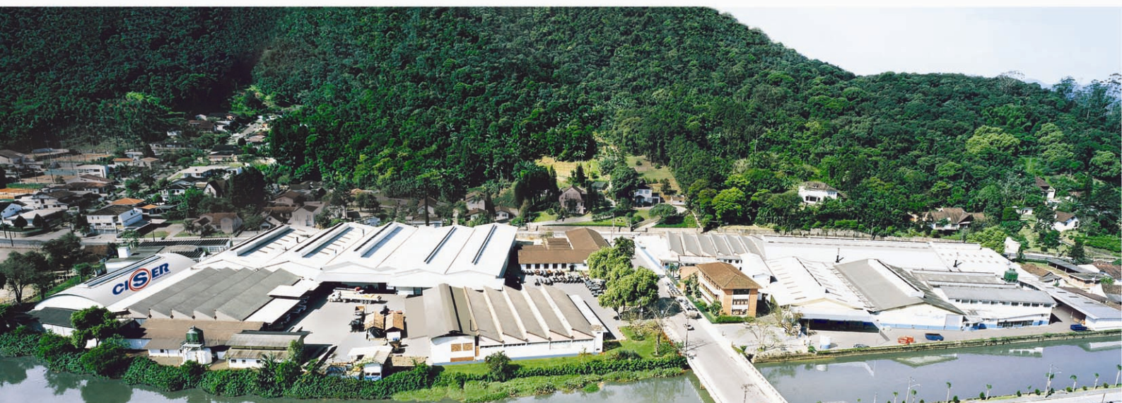
PLANTA INDUSTRIAL JOINVILLE SC
